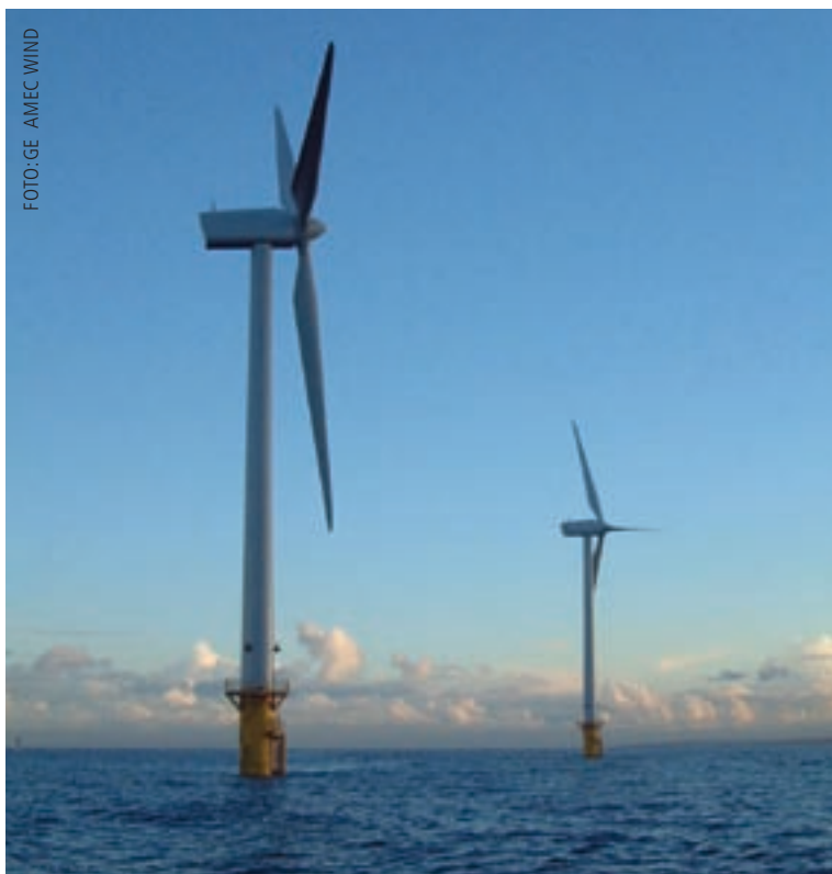
Blyth Offshore Generating.
